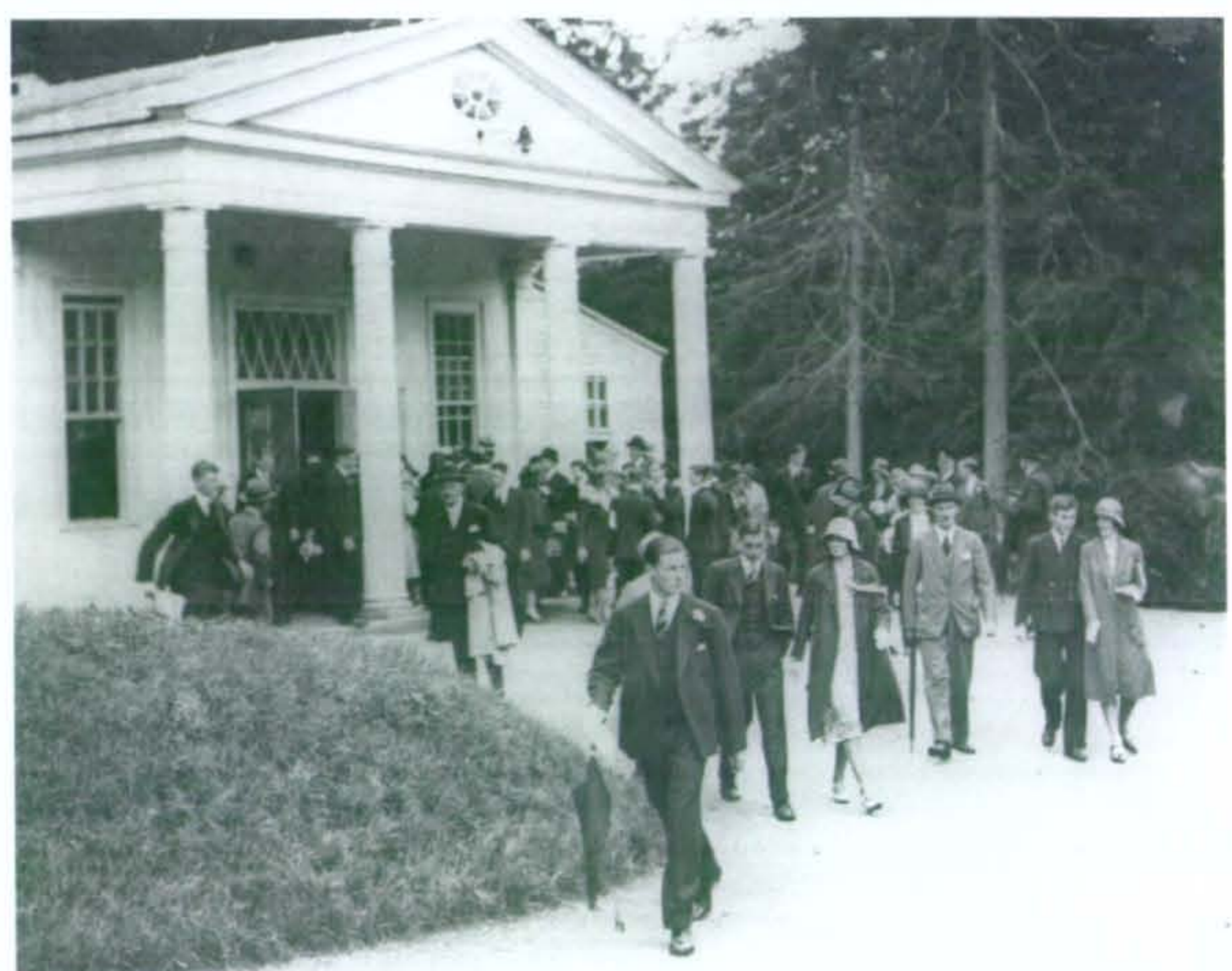
Below: The School's original sports hall, in the 1920s, a temporary structure designed by Clough Williams-Ellis.
