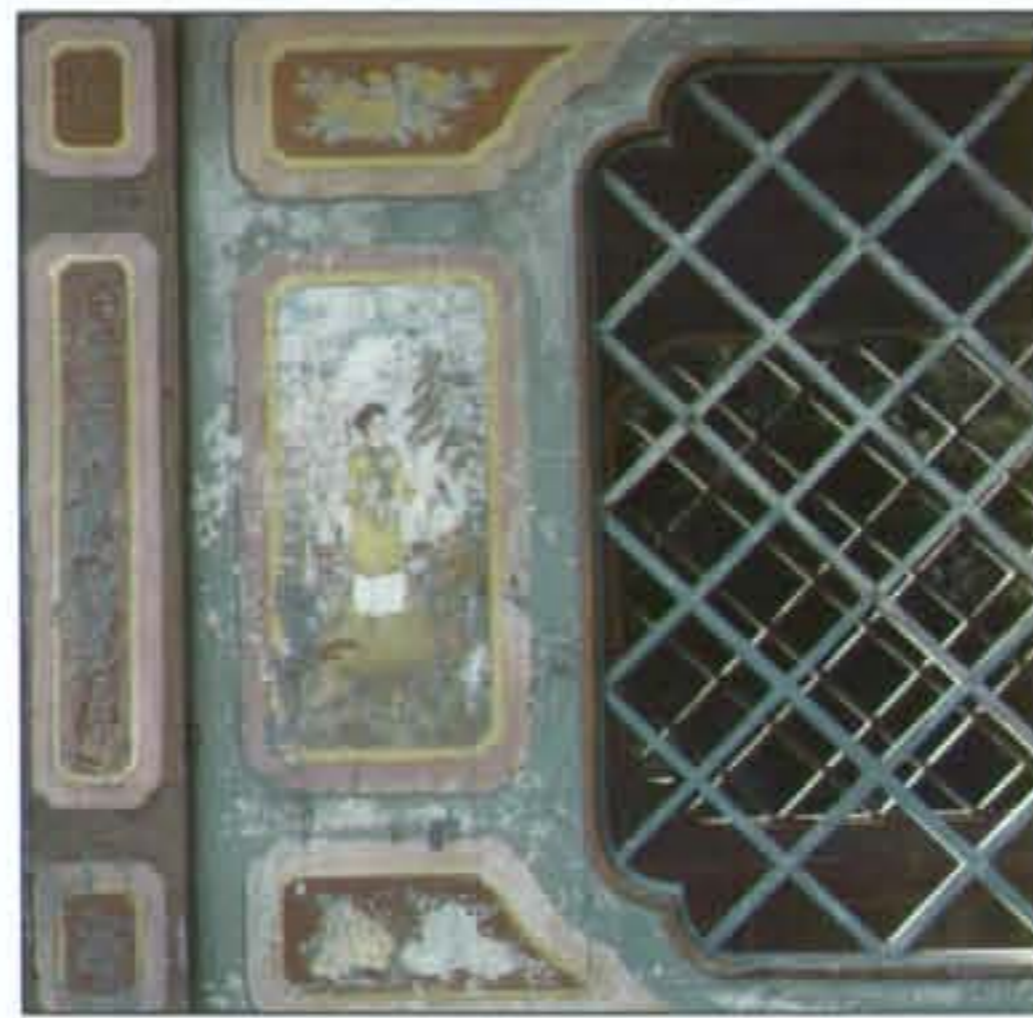
Painted details of the east side
