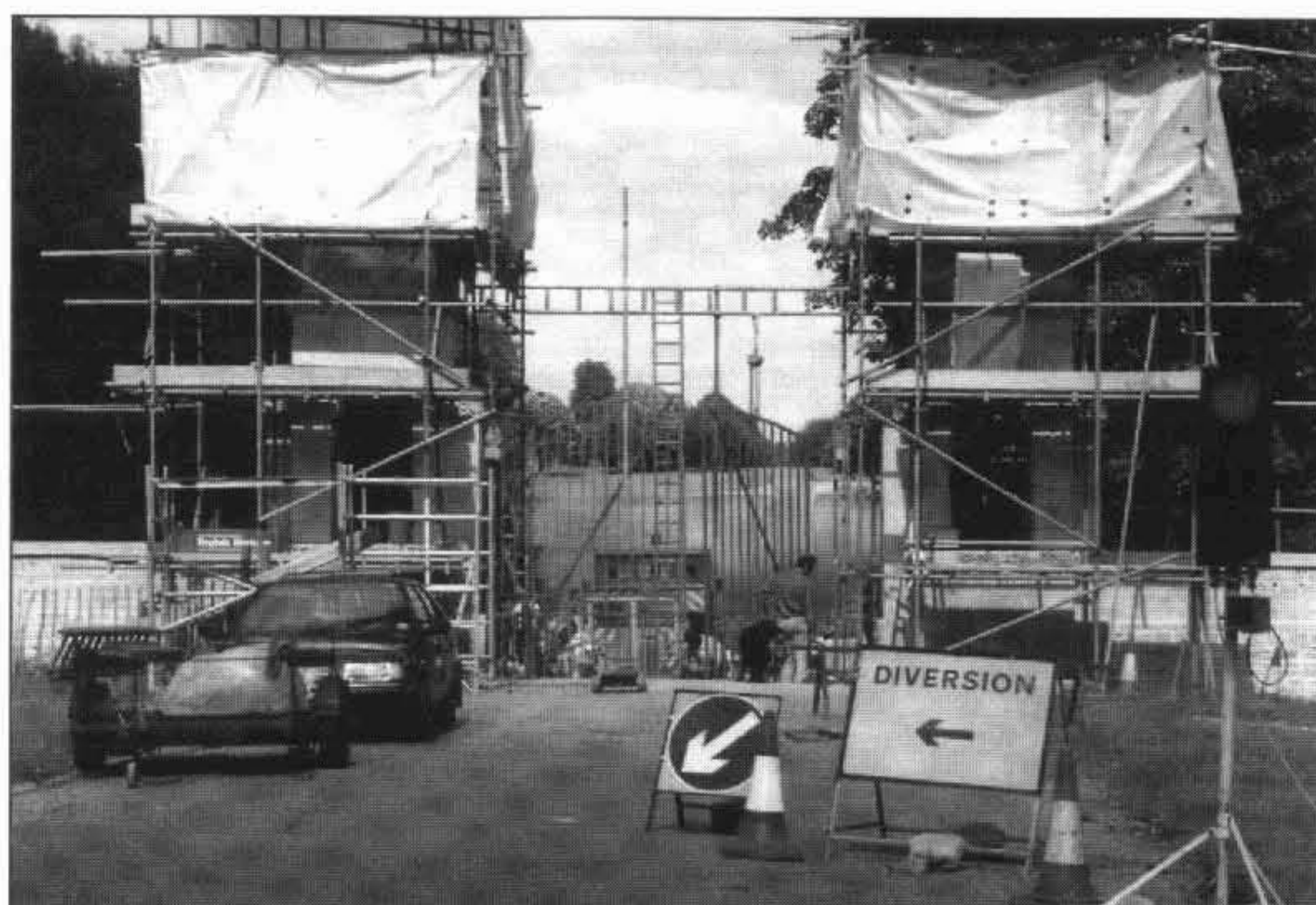
The new Oxford Gates being lowered into position
