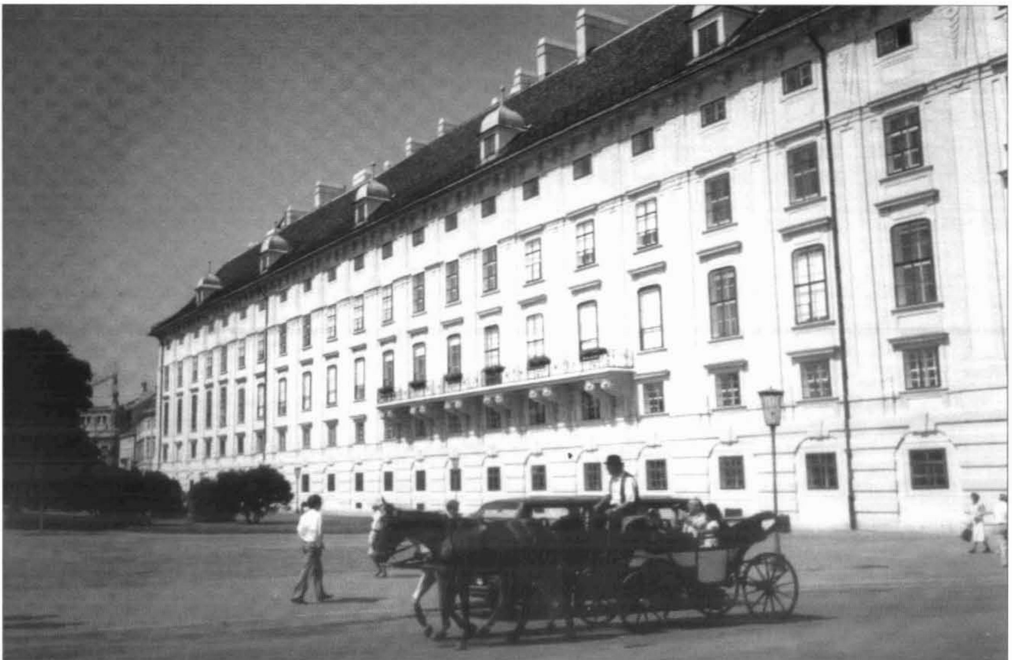
Vienna: Leopold's Wing, Hofburg Palace
