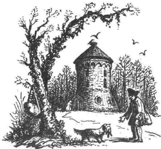
The Keeper's Lodge. Remodelled soon after 1800, it is now the Bourbon Tower.
